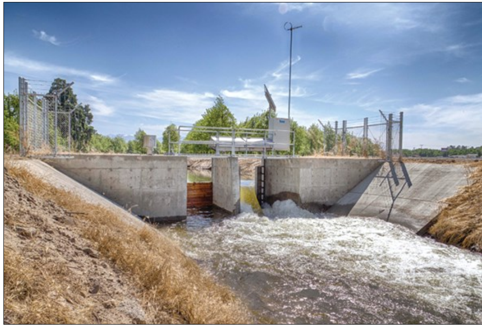
Figure 6-3. New Automated Check Structure in Packwood Creek
